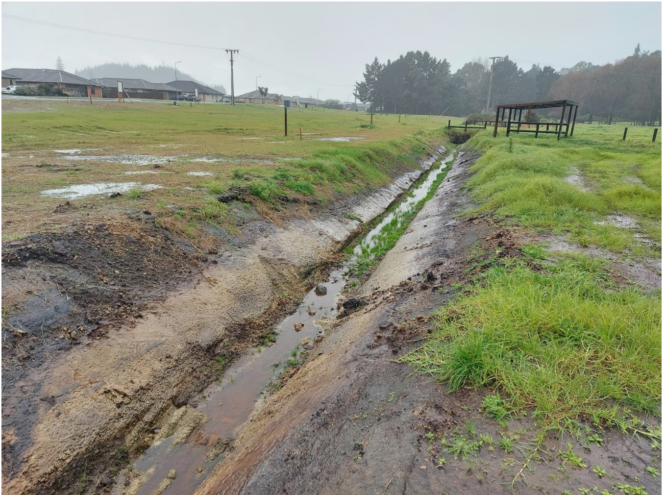
Figure 6: Exposure of the hardpan within a surface drain. Image taken looking approximately north on the western boundary of Lot 78.
